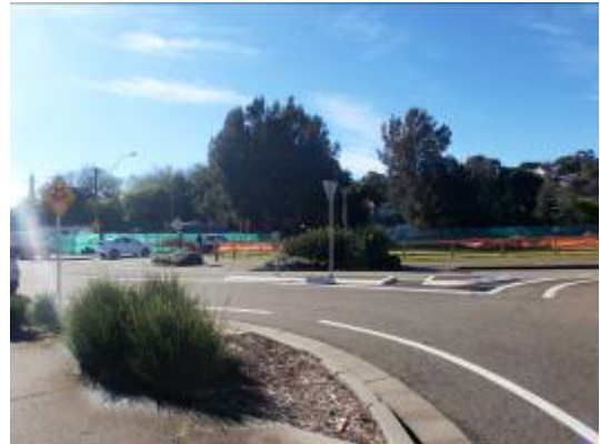
Figure 14 – Looking northeast to Nelson St and site access from The Crescent (from roundabout),
