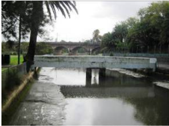
Figure 18 – Looking north to viaduct / light rail from Johnston's Creek Bridge.
