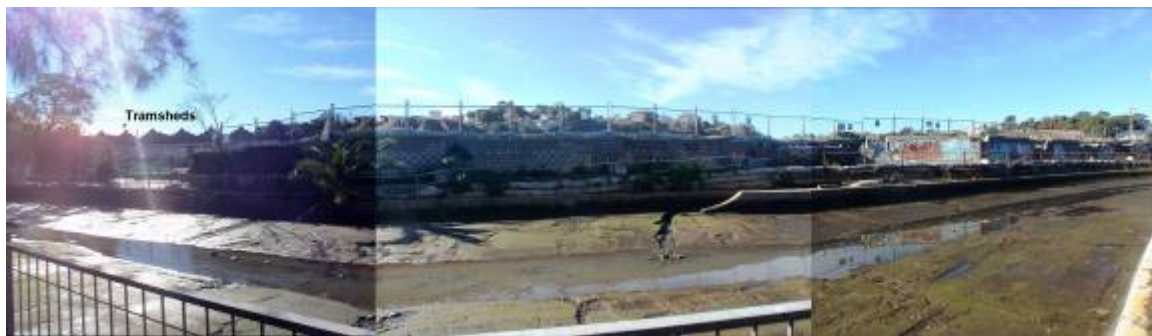
Figure 23 – Heritage listed former tram accessway and tram track fencing (handrail) along Johnston's Creek stormwater channel (looking east).
