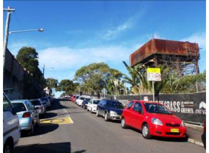
Figure 26 – Maxwell Rd, looking south. The Maxwell Road access will require the relocation of the heritage listed water tank.
