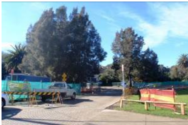
Figure 15 – Entry to Johnston's Creek Bridge from Nelson St / Chapman Rd.
