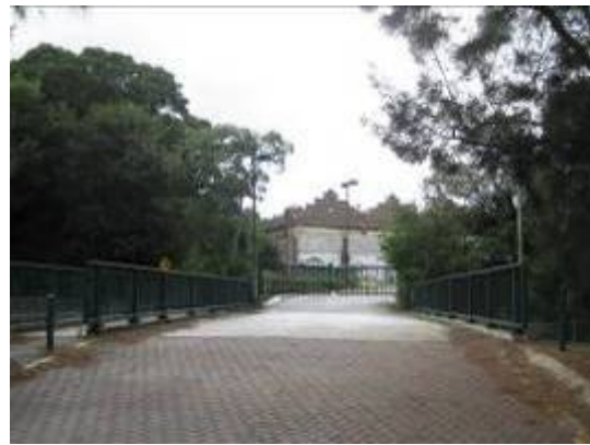
Figure 16 – Johnston's Creek Bridge. Tram Sheds in background.
